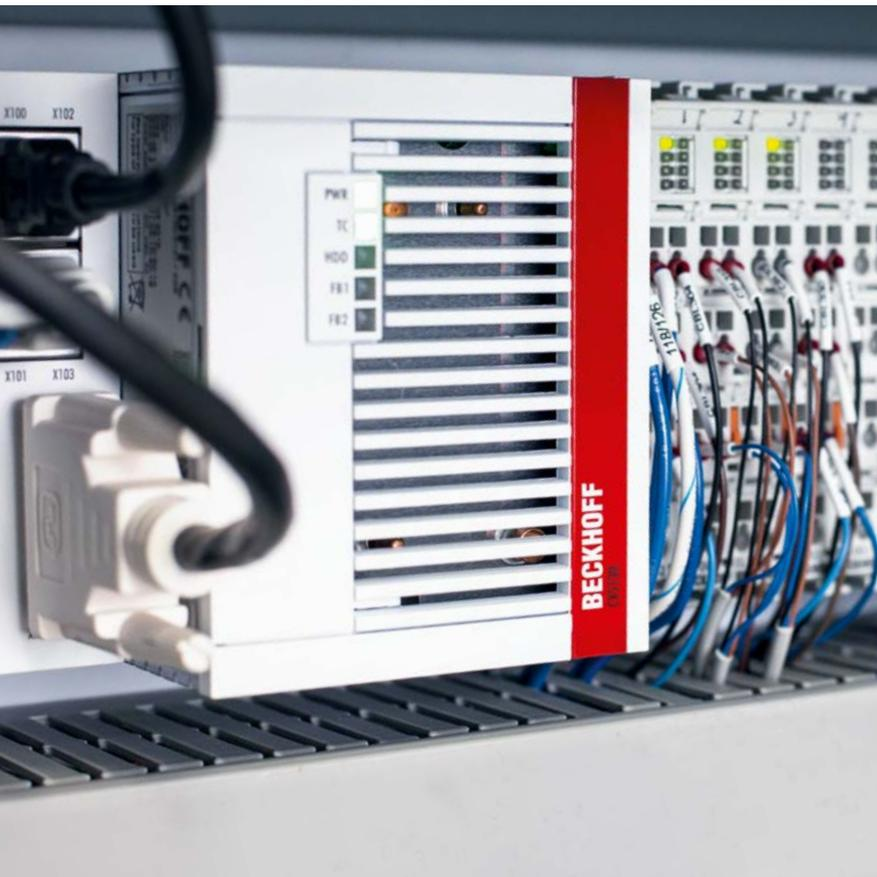
Itron uses the compact CX5130 Embedded PC from Beckhoff as its control platform.
