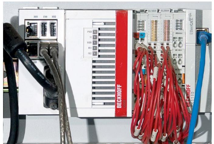
View inside the control cabinet of the CNC-800A3 with the CX5120 Embedded PC as the central control platform.
